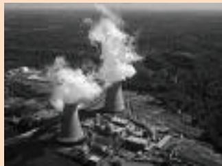
Cooling towers at Vogtle, near Augusta
