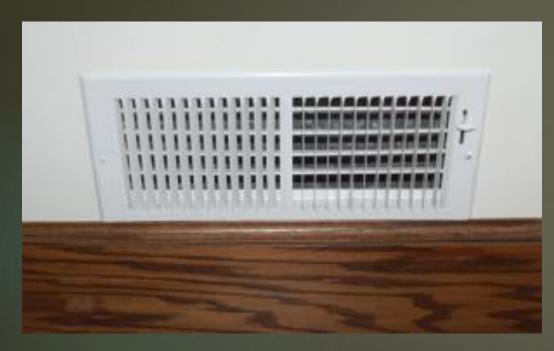
**PRO TIP:** Un-screw vent caps and clean them out thoroughly, removing dust and dirt to help air flow easily.
