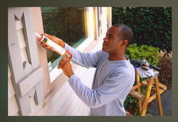
**PRO TIP:** Use caulk inside and out to make sure all cracks have been filled and no air can escape.
